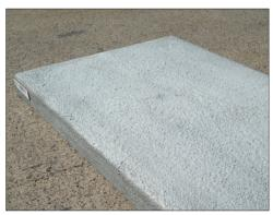
**STEP1**Position the lightweight slab in the required location of the ASHP unit.
